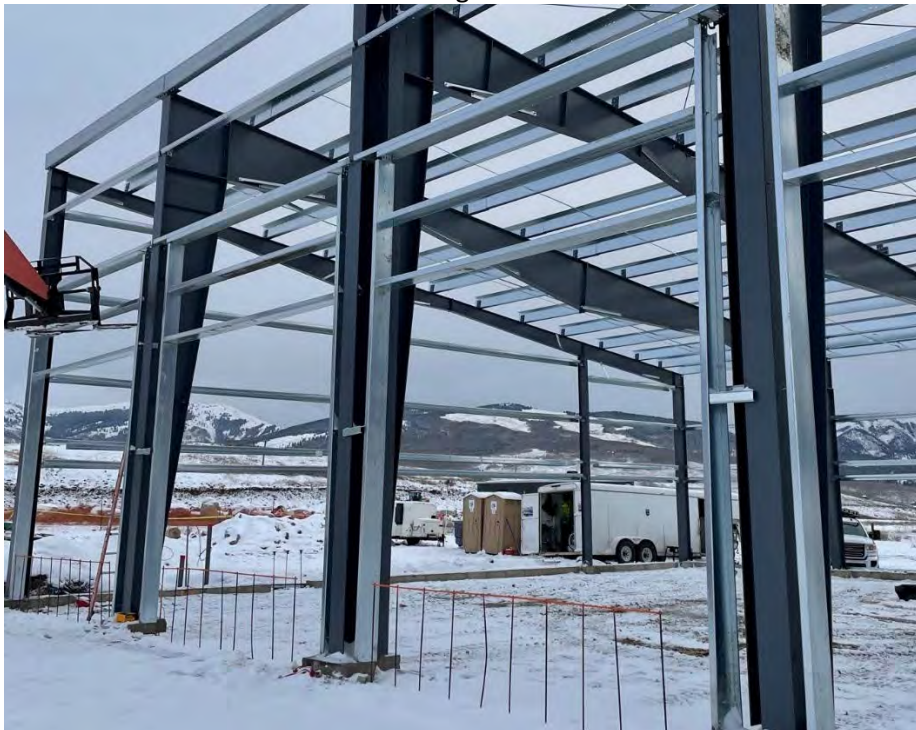
6. Secondary Steel and Detailing
