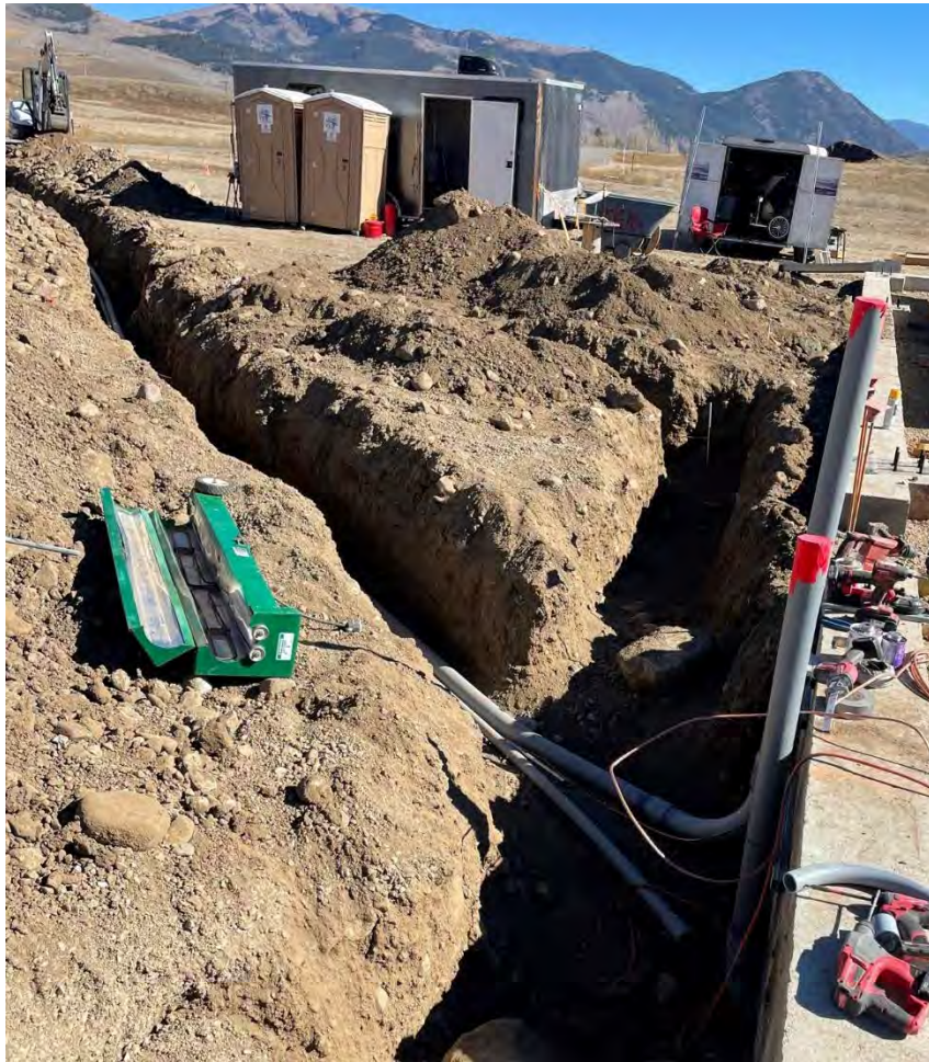
3. Exterior Electrical Underground
