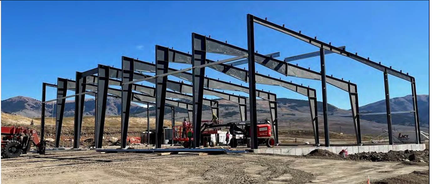
4. Primary Steel Erection
